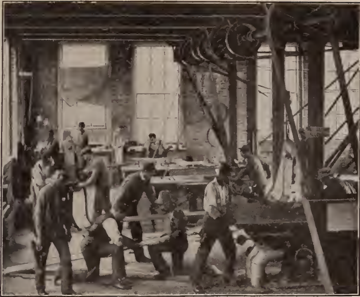
MANUAL WORK IN THE MEN'S INDUSTRIAL BUILDING AT BEREA
